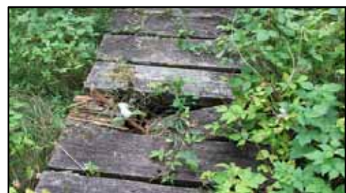
Above: Senkiw Swinging Bridge; middle: south side path to bridge; bottom: rotten boardwalk boards.
